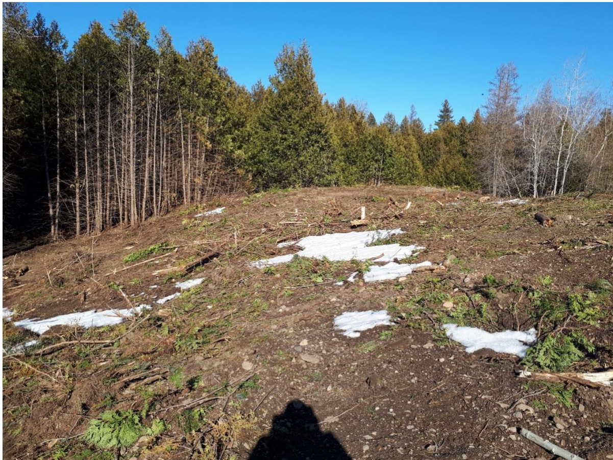
Photo 5. Looking East Tree Clearing
